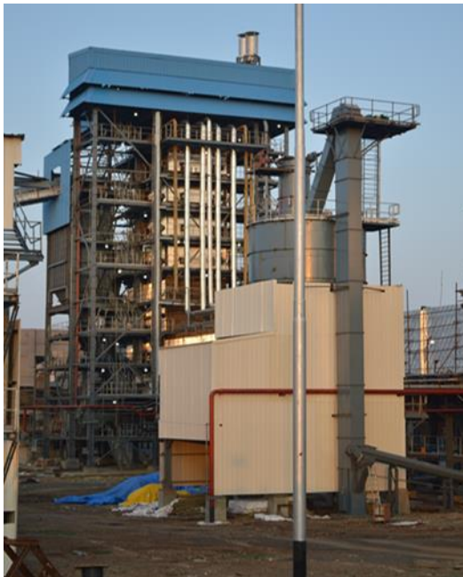
Incineration Boiler -40 TPH
